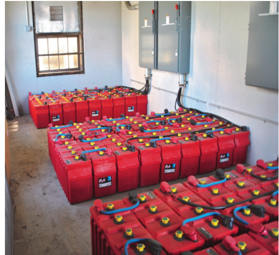
Fig. 2.3. A battery bank for an off-grid PV system on Georges Island in the Boston Harbor Islands.
